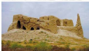
Going, going ... The 1400-year-old Little Kyz Kala fortress in Merv was in bad shape in 1950 (top); a rising water table accelerated the erosion, greatly diminishing the monument by 2003.
